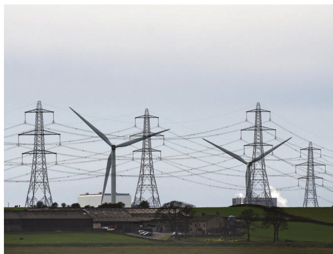
National Grid electricity transmission lines and pylons with wind turbines in Heysham, Lancashire, UK. Photo: Alamy
